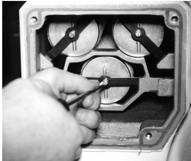
Fig. 3 - Removing Filter Spring
